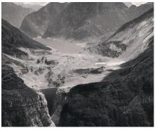
Figure 12.2 | An image of the Vajont reservoir shortly after the massive landslide (you can see the scar from the landslide on the right, and the dam is located in the foreground on the left). Author: Unknown Source: Wikimedia Commons License: Public Domain
