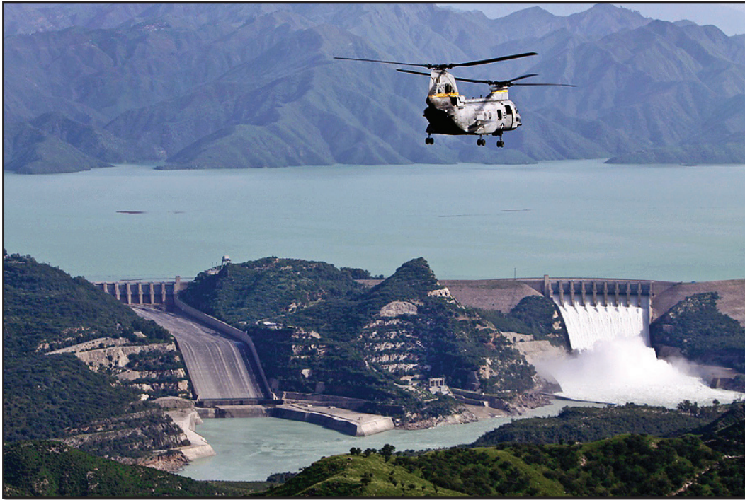
Figure 9.10 | World Bank Financed Tarbela Dam in Pakistan
