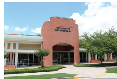
Figure 6.9: Cobb County government complex.
