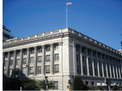
Figure 6.6: The United States Chamber of Commerce headquarters at 1615 H Street, NW in Washington, D.C.
