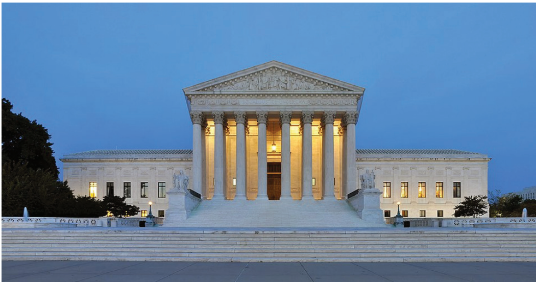
Figure 3.9: Panorama of the west facade of United States Supreme Court Building at dusk in Washington, D.C., USA.
